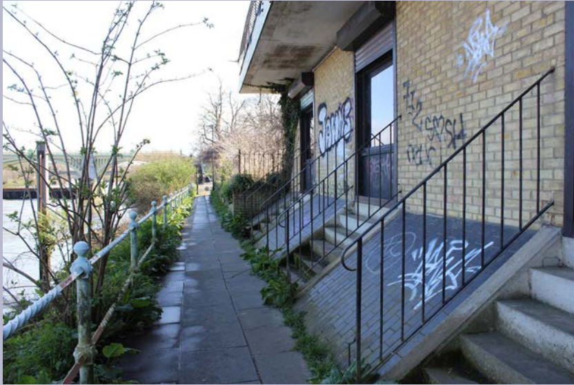
Existing photo of the unwelcoming environment of the footpath, showing the area which currently attracts anti-social behaviour.
